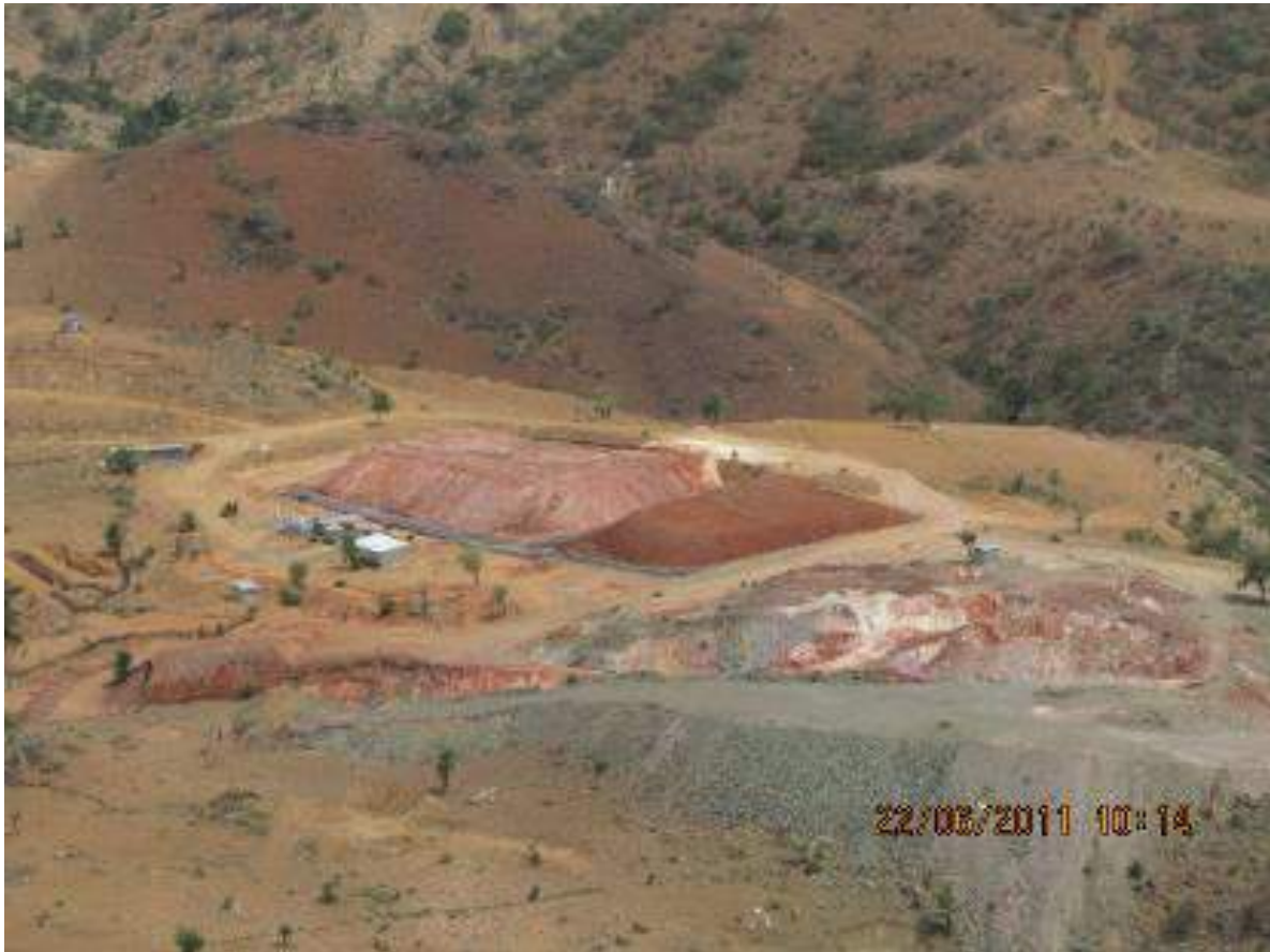
Photo 6-3 Mai Argab zone, 5,000 tonnes of stacked heap leach oxide material
